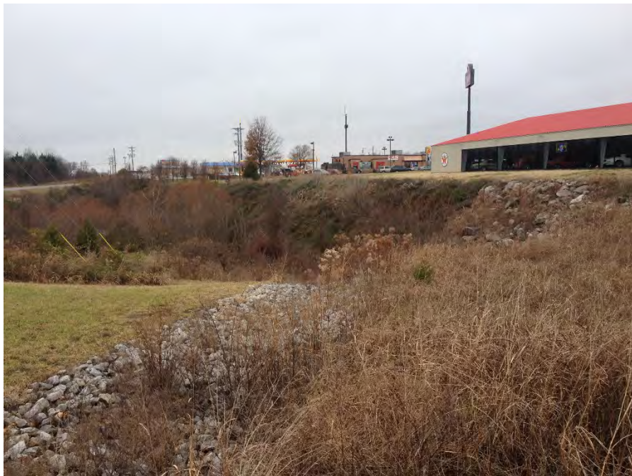
Figure 7-Sinkhole behind Art's Corvette showing significant relief with crushed stone lining drainage ditch
