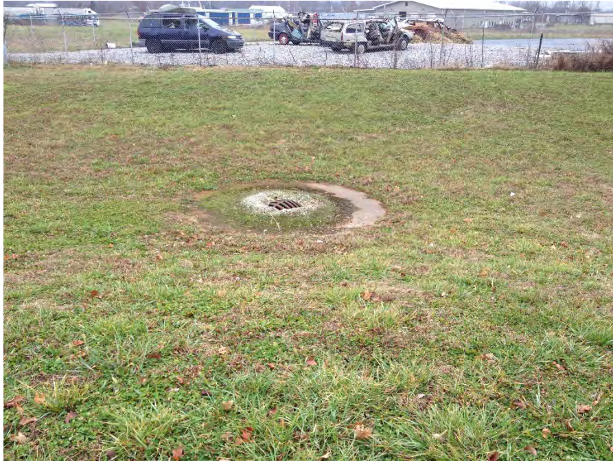
Figure 6-Drywell installed in Sinkhole Depression off Parker Drive
