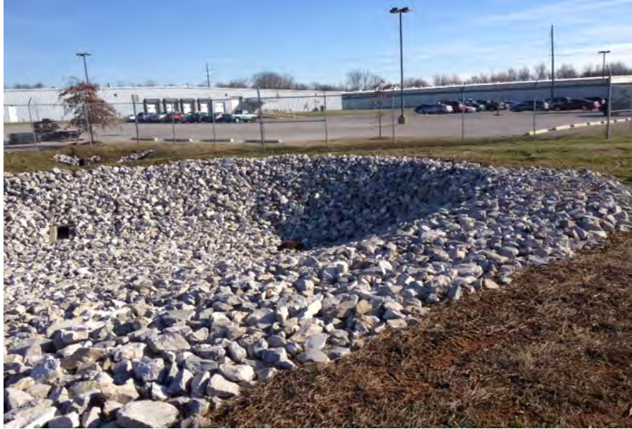
Figure 8- Lined surface depression utilized for drainage in commercial area
